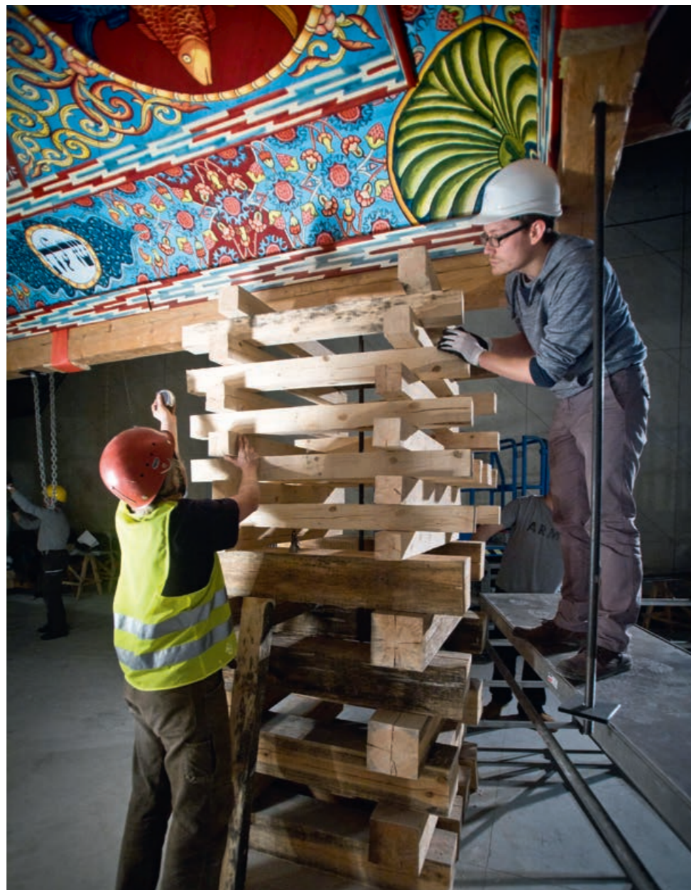
— Installation of the replica of the Gwoździec synagogue roof, March 2013
