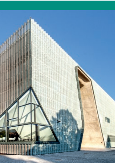
Supporting POLIN Museum’s activities by carrying out joint projects
